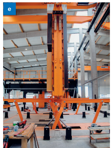
Fig. 9c-e: Two Abus indoor cranes, each with a load capacity of 12.5 tonnes, lift the prepared butterfly formwork until the backs of the two formwork panels touch (the prepared formwork panels face outwards).
