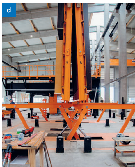
Fig. 9c-e: Two Abus indoor cranes, each with a load capacity of 12.5 tonnes, lift the prepared butterfly formwork until the backs of the two formwork panels touch (the prepared formwork panels face outwards).
