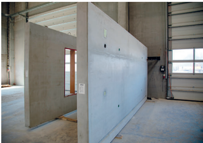
Fig. 11: Freshly demoulded walls - with the exception of the filling side, all five sides and the edges and surfaces of the recesses are absolutely smooth.
