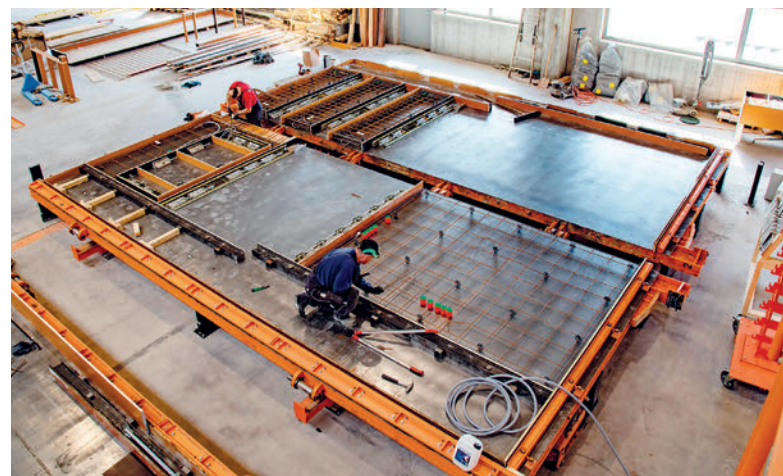
Fig. 7: View from the side catwalk of the battery mould down to the two work stations with the butterfly formwork lying folded out – on the right-hand panel of the completely visible butterfly formwork, the shuttering for three columns for the interior of a building is visible.
