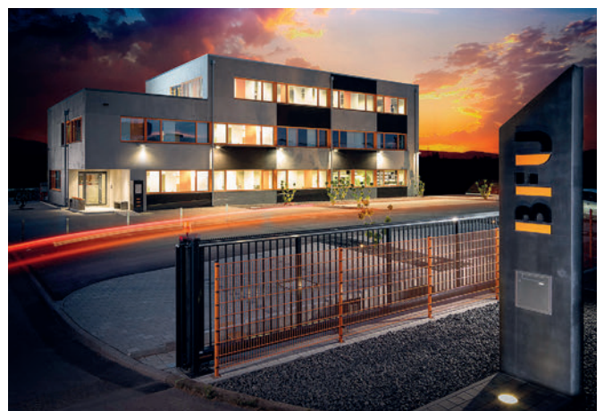
Fig. 2: The BFU headquarters in Schramberg-Waldmössingen was built in 2013 - of course using precast concrete elements from the company's own production.
